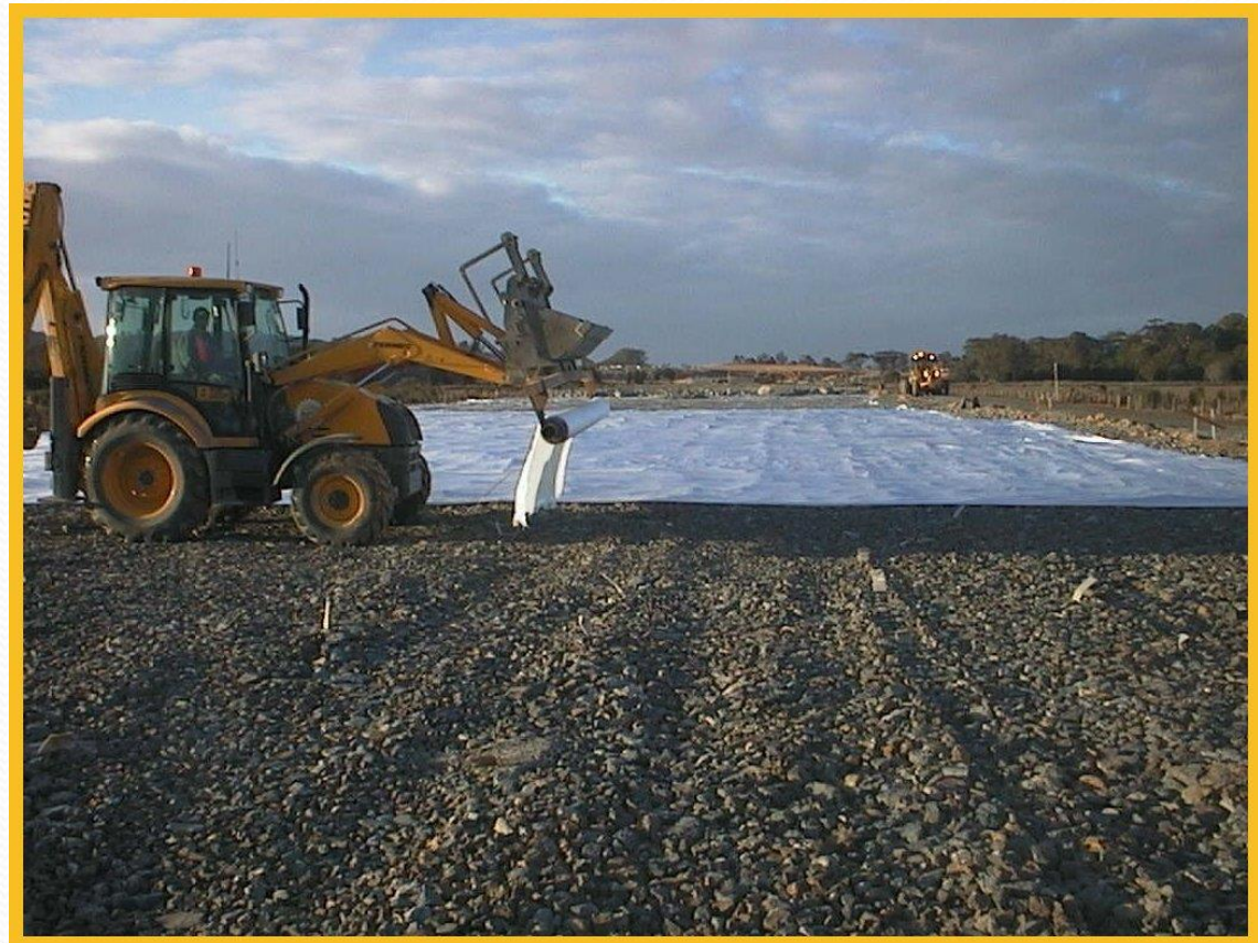
Geofabrics used on Pacific Highway
