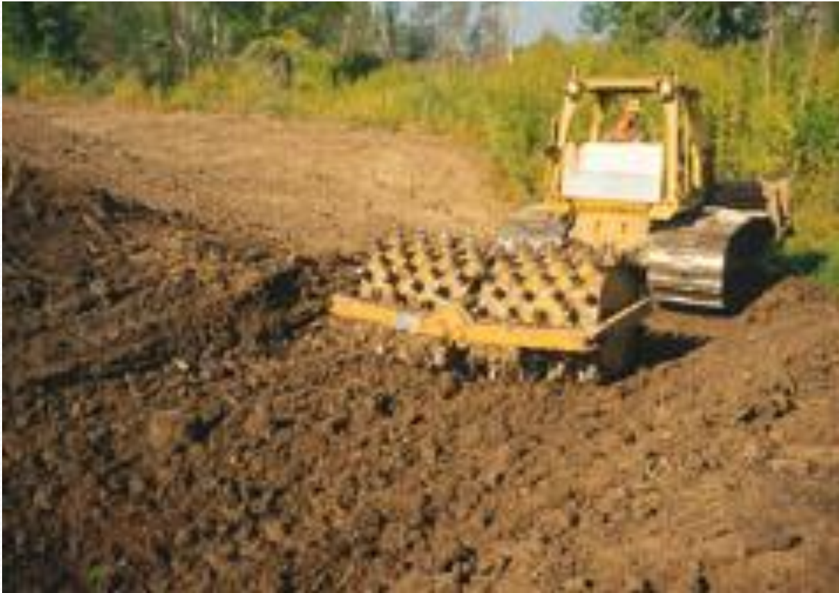
Sheepsfoot Roller to Compact Clay Soils
