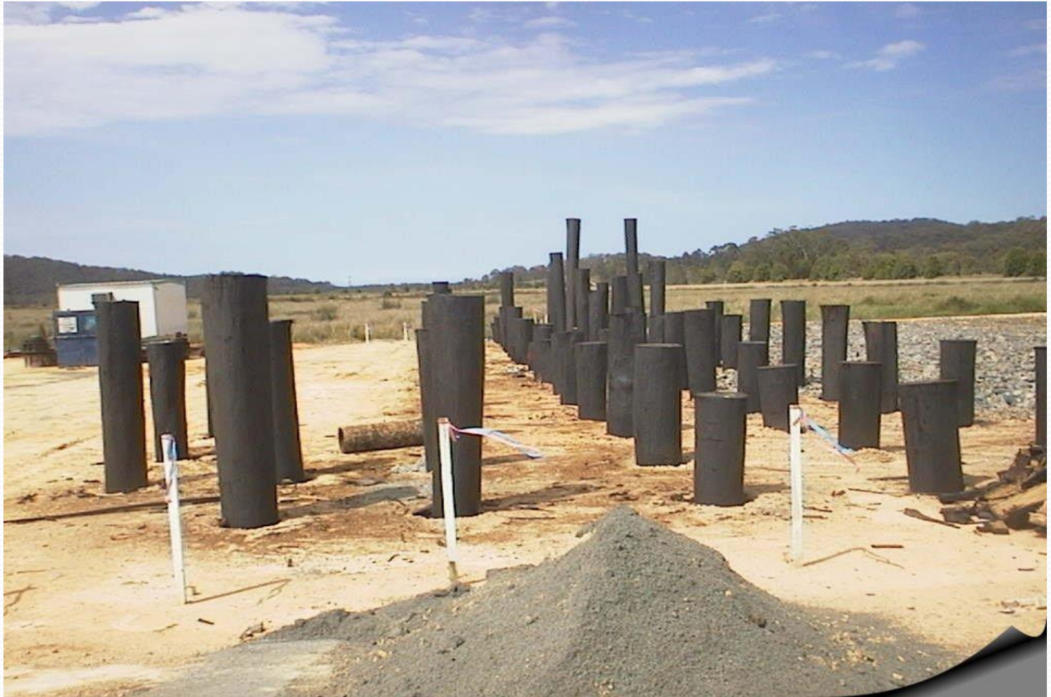
Driven timber piles, Pacific Highway
